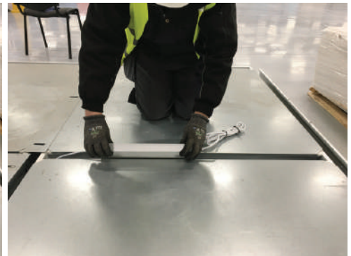
Carefully insert gear encloser into noggin
