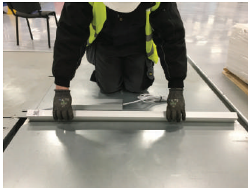
Seperate gear enclosure and insert Luminaire into noggin
